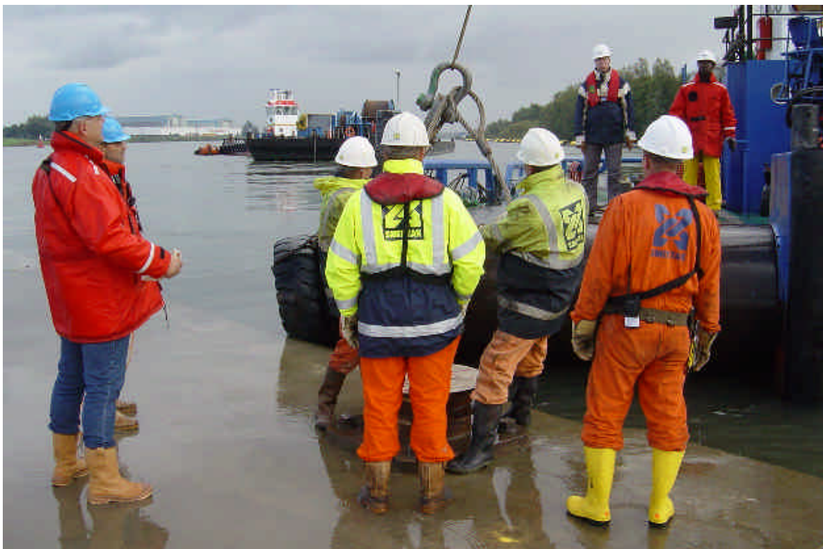
Saturday the 5 th element of the newbuilding HSL tunnel under the Oude Maas was transported by 4 tugs and 1 pusher tug from Barendrecht to final location
