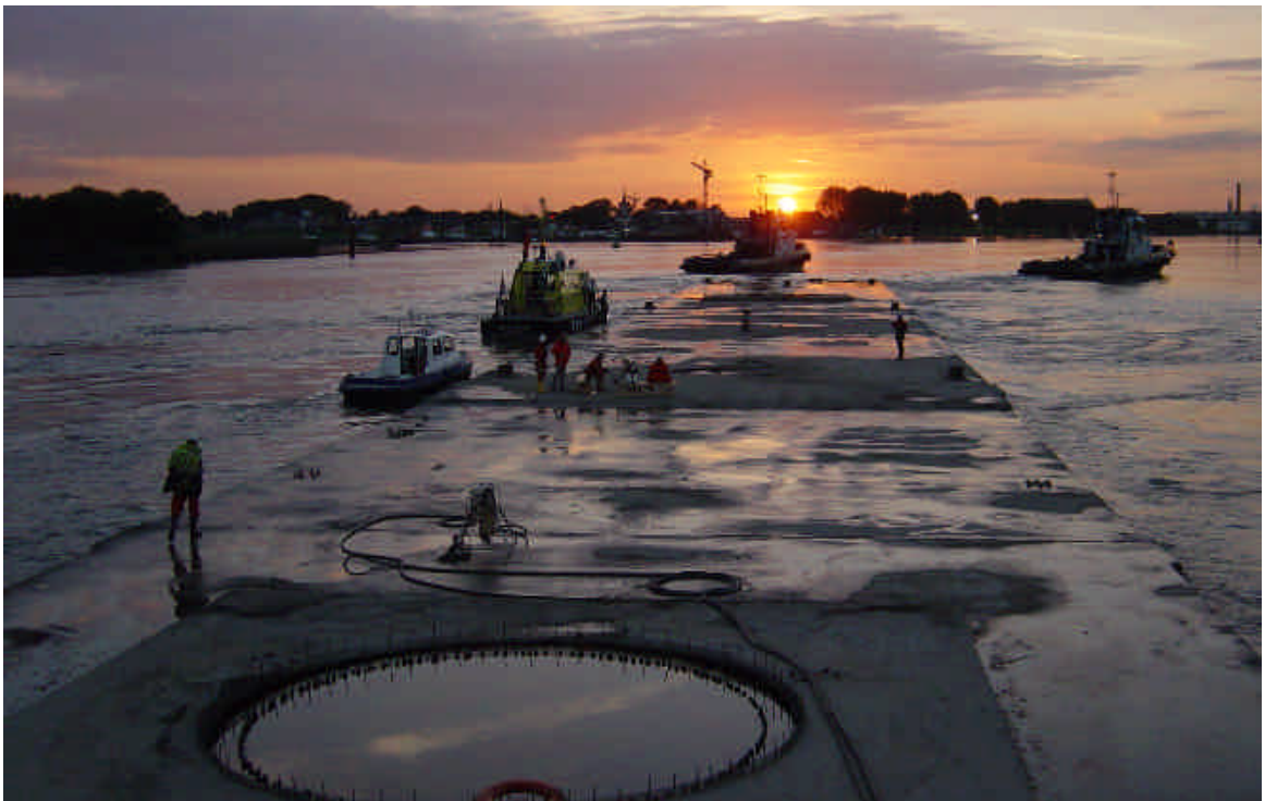
Saturday afternoon/evening 4 tugs and 1 pusher tug transported the 4 th element of the Oude Maas HSL tunnel from the building site to the installation site
