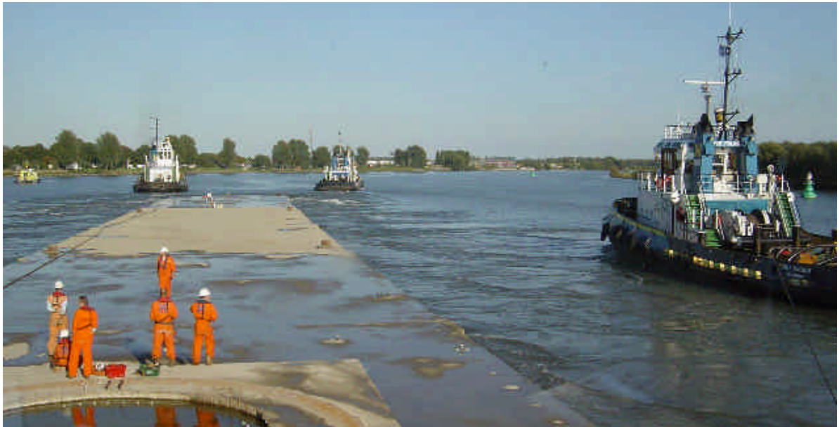
Saturday afternoon the second part of the new to built HSL tunnel under the Oude Maas was towed from the building dock in Barendrecht to the installation site in Zwijndrecht
