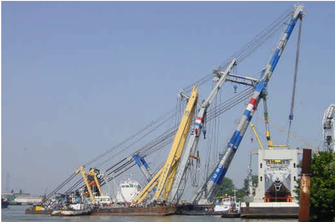
Smit had a heavy lift job at Kinderdijk. On the photo the 1500 tonnes weighing cutterladder hanging in the tackles of the Taklift 3 Matador 2 & 3 , during the installation into the dredger JF.J de Nul .
