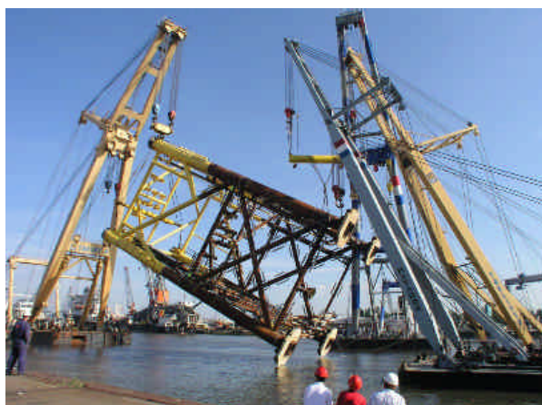
Taklift 4 and Taklift 3 and Matador 3 and Matador . The 1100 tonnes Shell -CARRACK jacket, which was build by HBG from Schiedam,
