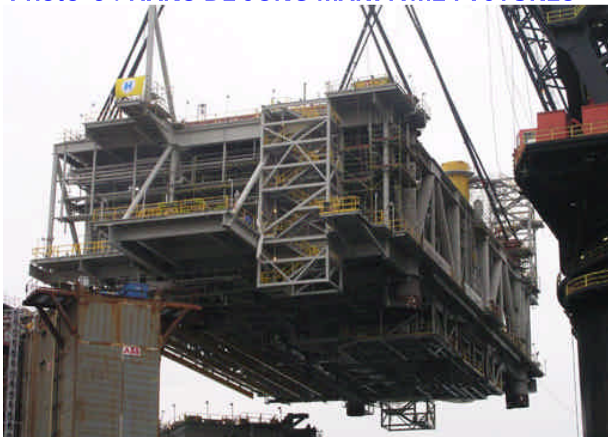
Offshore Crane vessel Thialf , moored at Caland canal Europoort, installing the 2nd module with the two powerfull cranes on the TLP which is build to operate in the future in Angola. The weight of the 2nd module was almost 6000 tonnes
