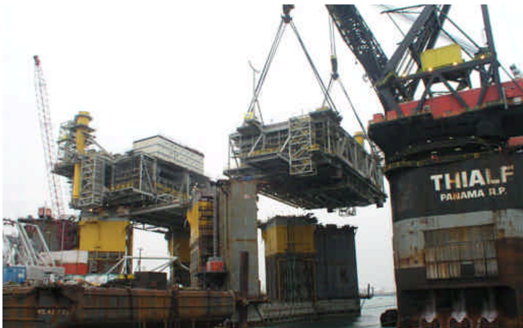
Offshore Crane vessel Thialf , moored at Caland canal Europoort, installing the 2nd module with the two powerfull cranes on the TLP which is build to operate in the future in Angola. The weight of the 2nd module was almost 6000 tonnes
