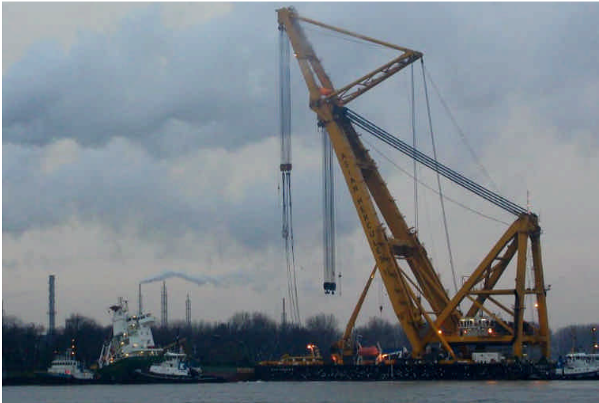
The Sheerlegs ASIAN HERCULES II connecting the lifting slings to the Western Trader . Photo : Aad Horiens ©
