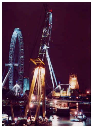
Due to operational constraints, the lifts were performed in two stages. Between 2100 and 2300 hours, Taklift 3 lifted a pylon element from a barge and rotated it into the installation position. Between 0030 and 0430, the sheerlegs manoeuvred with the element in its hooks to the installation site for final positioning on the bridge line.
