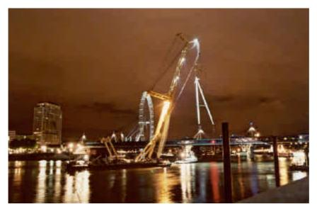
During the early hours of May 20, SMIT commenced the final phase of its involvement in the construction of two new pedestrian foot bridges spanning the River Thames, located on either side of the existing Hungerford Bridge. SMIT's floating sheerlegs Taklift 3 called at London for a six day visit to perform a series of lifts for the installation of six pylons for the downriver crossing. These are four stand-alone pylons, each weighing 30 tonnes; a 42
