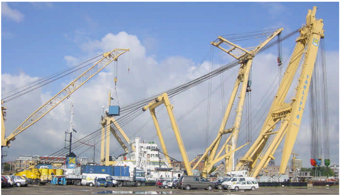
The Taklift 4 which returned in Rotterdam from the Monaco pier extension project is offloading the project materials in the Schiehaven in Rotterdam - Photo : Piet Sinke ©
