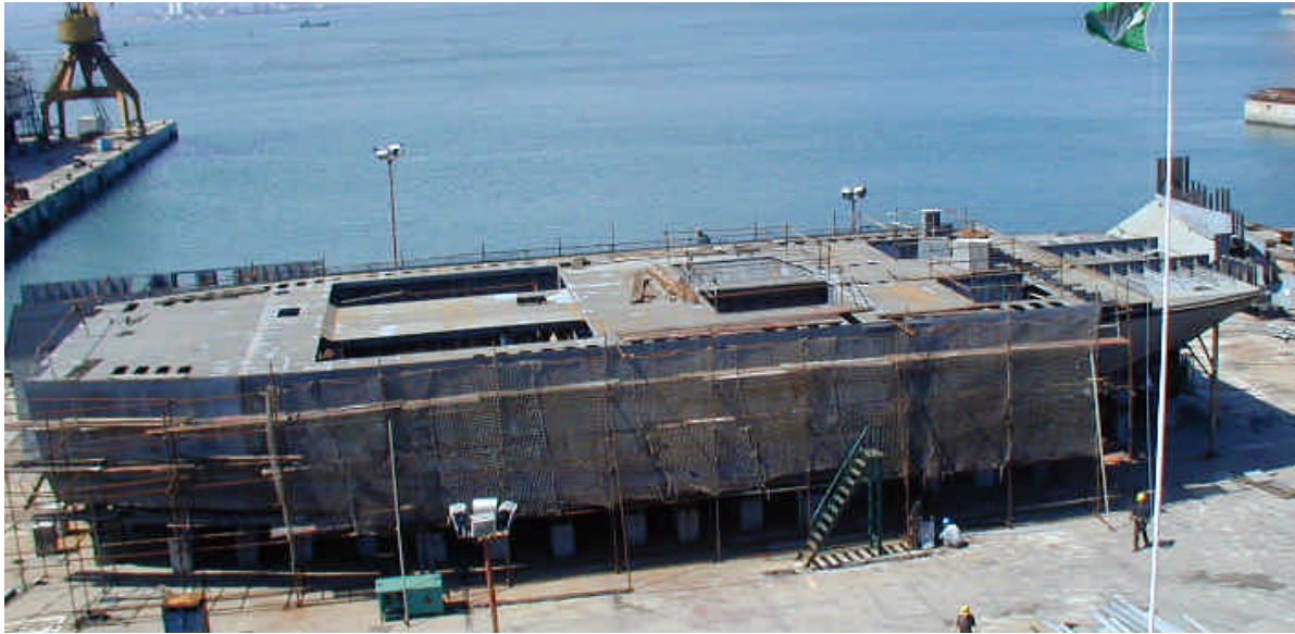
The ANGLIAN SOVEREIGN under construction at the Yantai Shipyard photo : Bill Davidson © – Klyne Tugs
