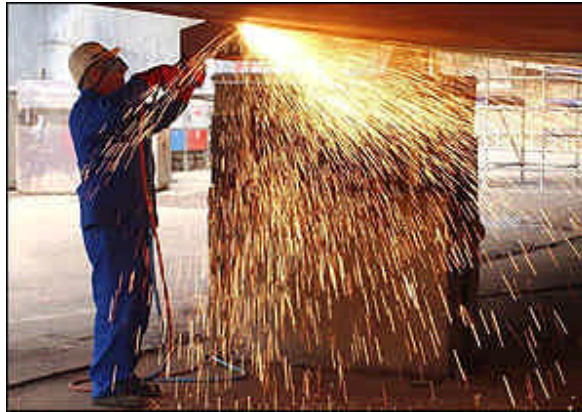
Sparks fly ... work is under way
