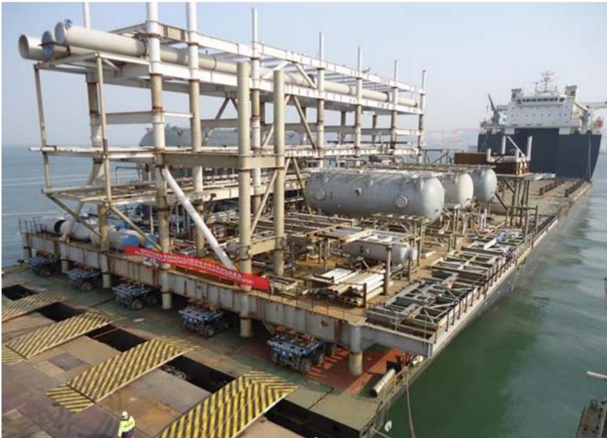
In the port of Qingdao (China), heavy lift vessel RED ZED II is ready for the SPMT load-out of a LNG plant module
