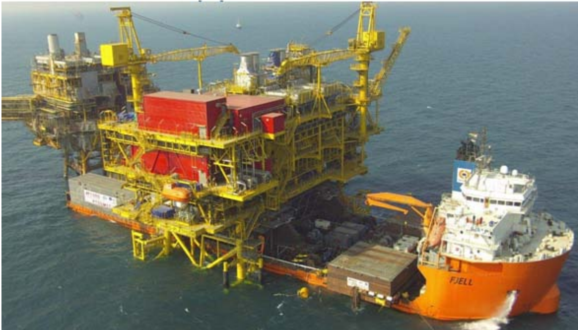
Nice drone picture of the HRD platform project where the topside was successfully installed by float-over method on 15-January by the FJELL photo : via Koen Brouwers
